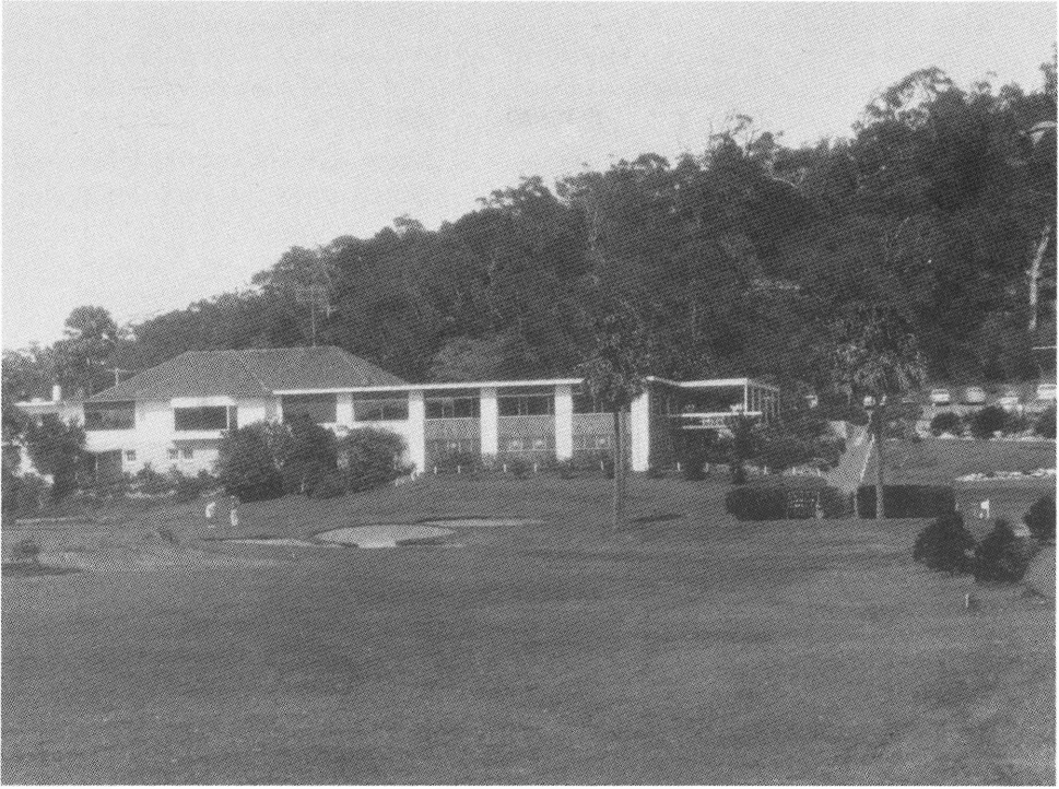
The Second Clubhouse Extension.
