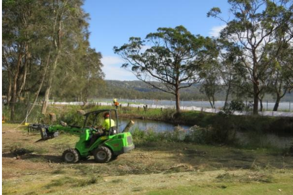
Figure 8 Construction of the new 15th hole
