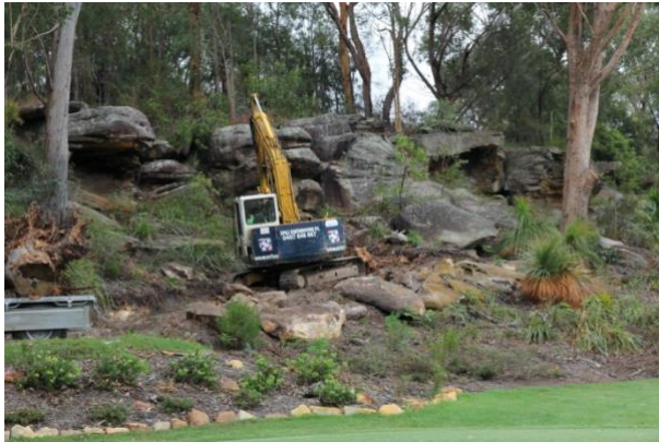
Figure 4 Path construction behind 13 th green
