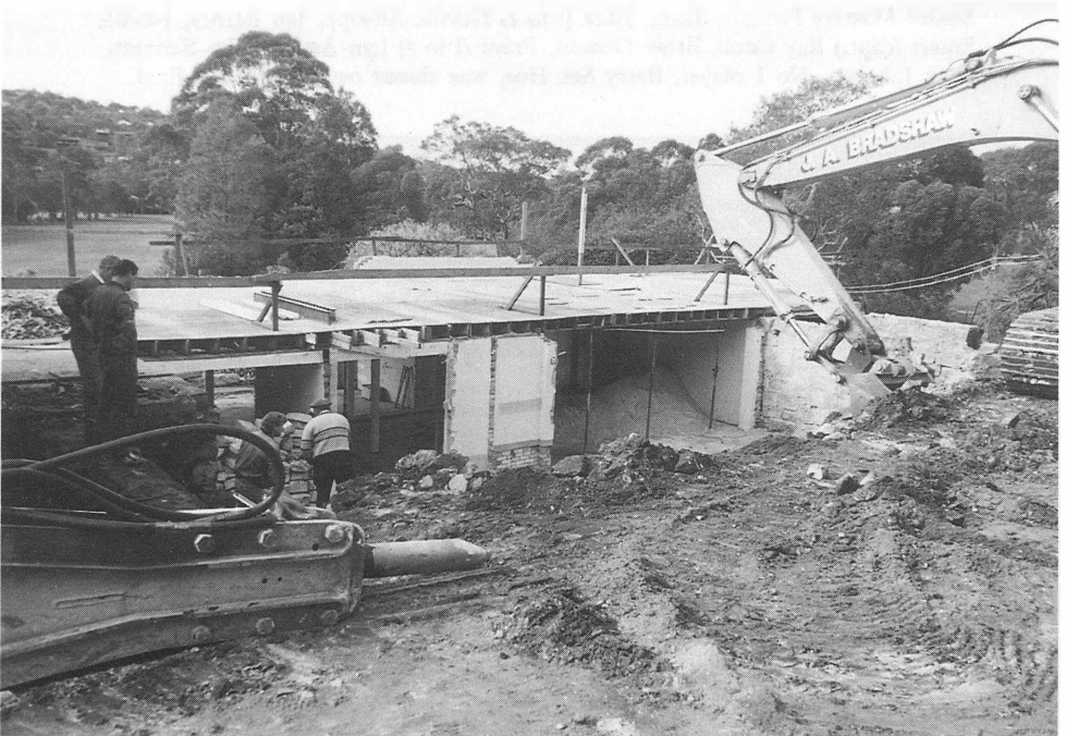
The walls come tumbling down.
