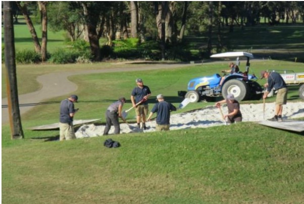
Figure 5 New bunker on the 8th hole
